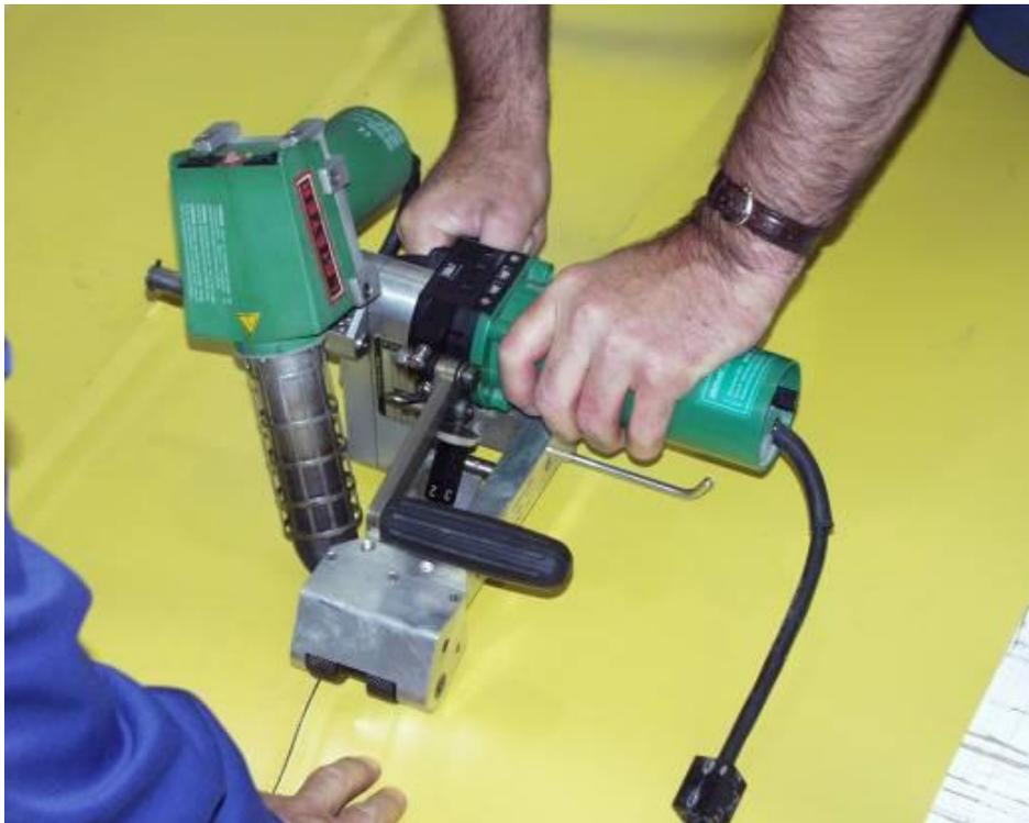
Heat welding with automatic welding machines (double seam) – welded seams as strong as the membrane
