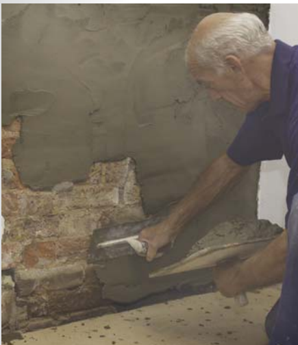
Render Coat Sand and cement with DryWall salt retardant additive
