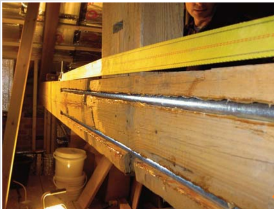
Repairing fractured roof truss tie beam
